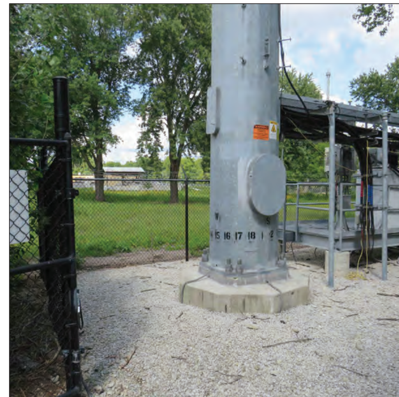
5 EXISTING TOWER BASE SCALE: NOT TO SCALE
