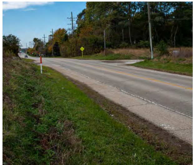
Existing site access to Subarea 1 and Subarea 2 on Klasen Road.
