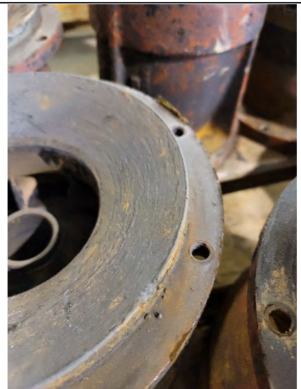
Mating bowl faces are deteriorated due to graphitization
