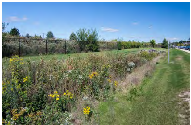
A parking lot at the Morton Arboretum features permeable pavers and bioretention islands (top) and a vegetated swale filters runoff from a parking lot in Aurora, IL (bottom).
