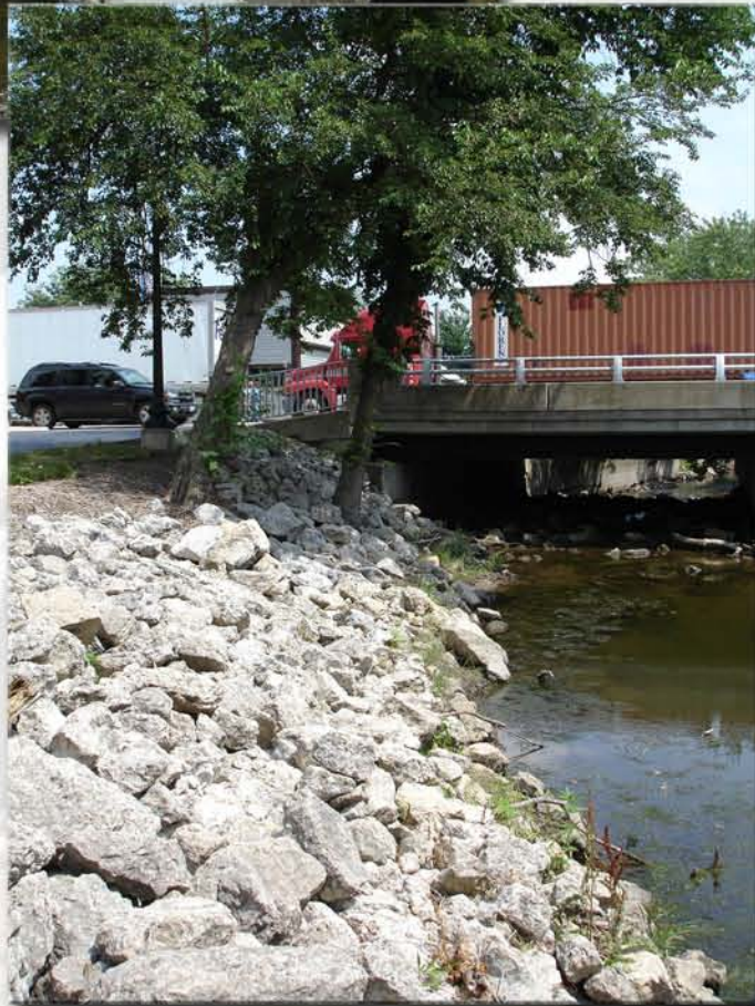
B. Southeast at Creek's edge
