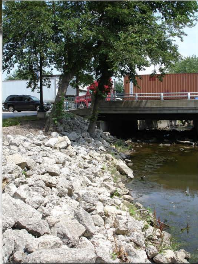
B. Southeast at Creek's edge
