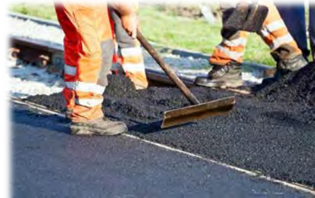
repairing and resurfacing Village streets for improved travel
