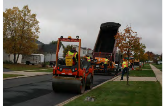
Resurfacing work performed on a residential street in Algonquin
