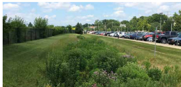
A bioswale used to control stormwater runoff near Metra's Aurora Transportation Center.
