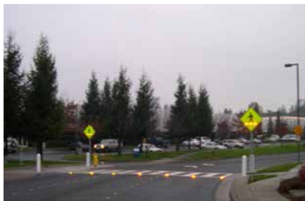
Photo of an improved pedestrian crossing consisting of an automatic bollard light activation and LED enhanced pedestrian crossing signs. Location is at the Cisco System Campus in California. Source: snipview.com.
