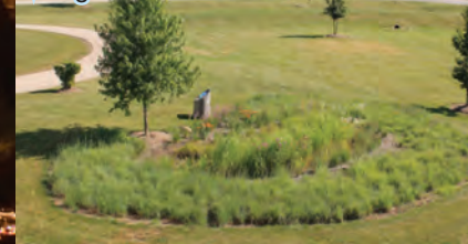
Rain garden infiltrates runoff before it discharges to the stormsewer at Village Water Treatment Plant
