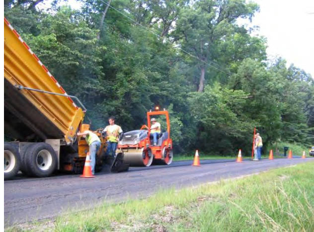
Village crews paving Highland Avenue
