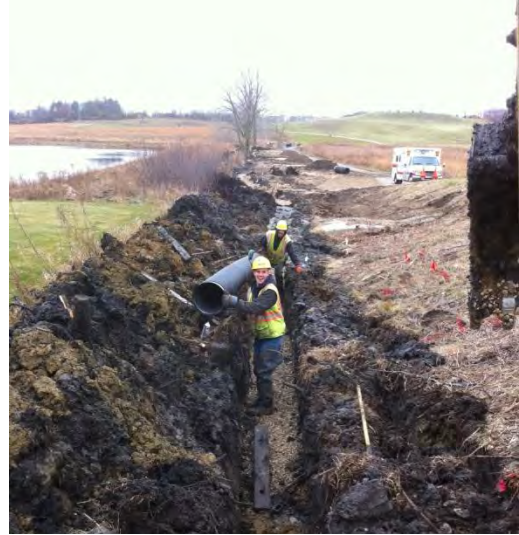
Village crews installing storm sewer drain
