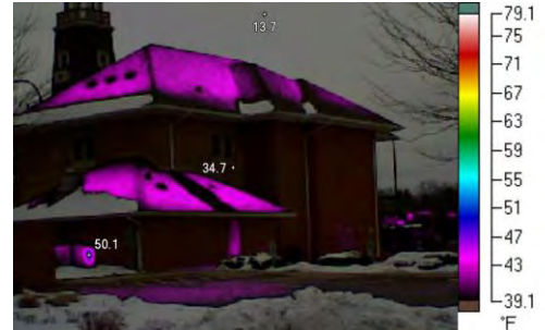
Thermal Image of Historic Village Hall identifying heat loss, provided by the Internal Services Division.
