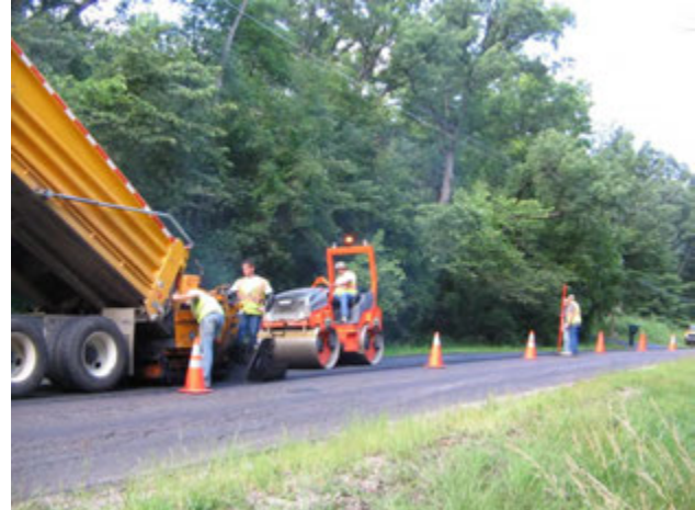
Public Works Department repaving Village roadway
