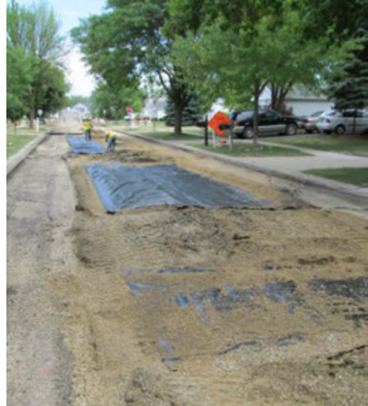
Arrow Road Construction repairs subbase in Spring Creek Subdivision
