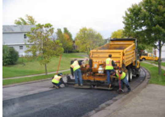
Streets crews work on installing a manhole
