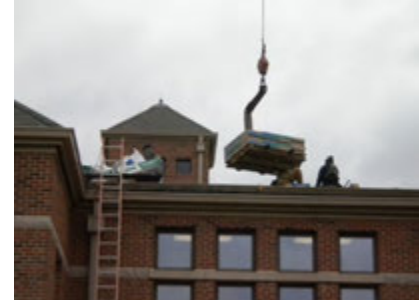
Ganek Municipal Center Roof Replacement
