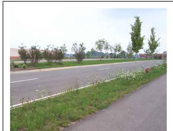
Completion of the Corporate Parkway Trail is ongoing as development of the Algonquin Corporate Campus progresses.
