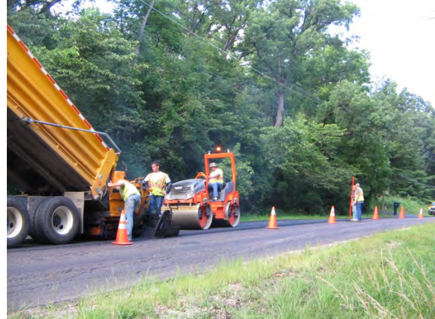
Public Works Department repaving Village roadway
