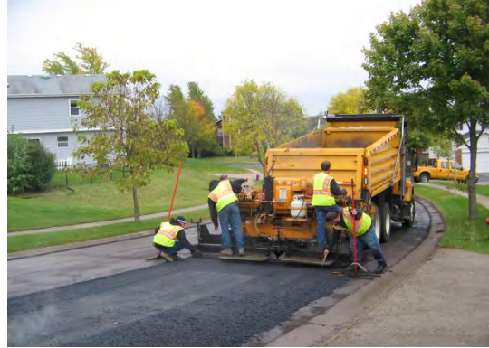
Streets crews work on installing a manhole
