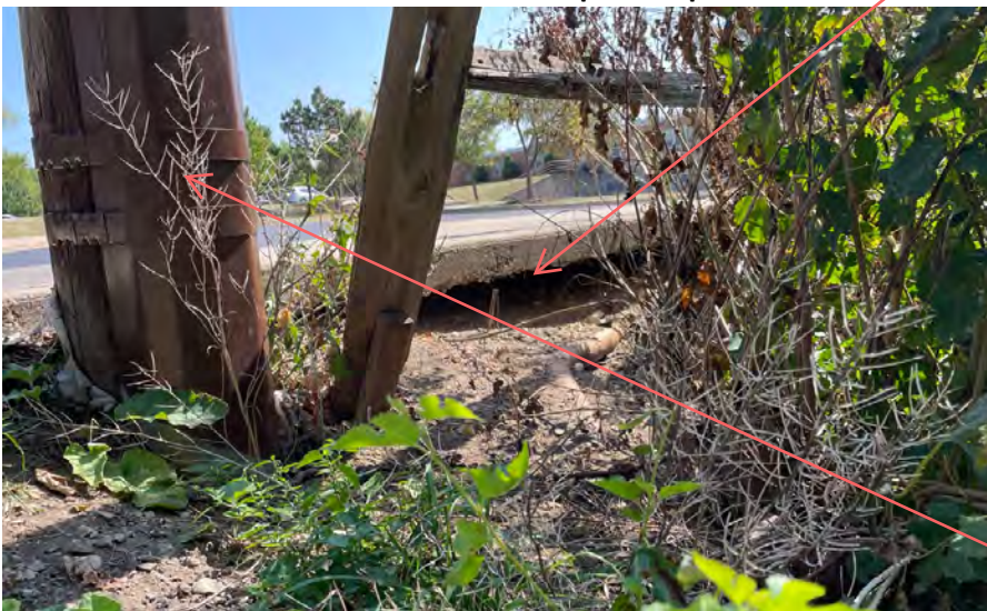
Photo 3 - Erosion causing undermined sidewalk & dangerous conditions
