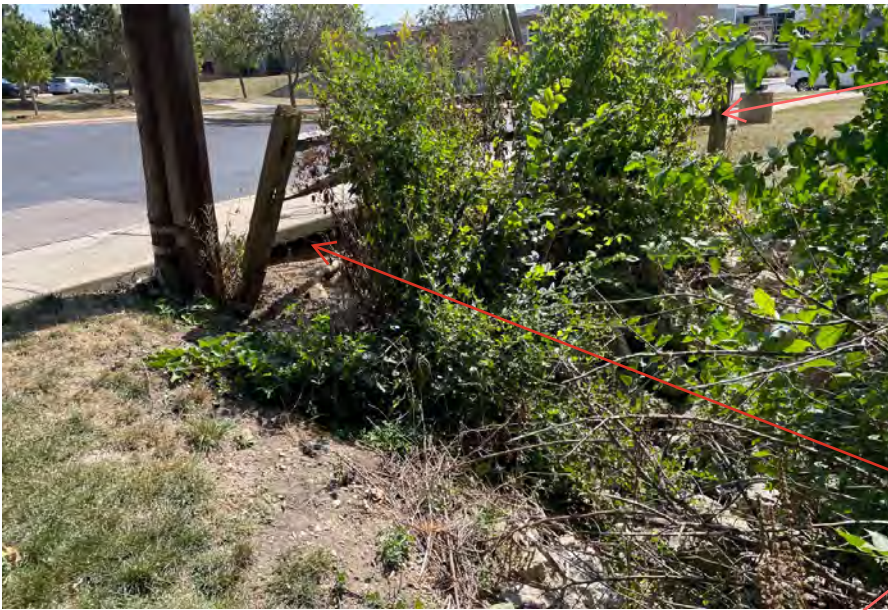
Photo 2 – Undermined sidewalk at ComEd pole in question
