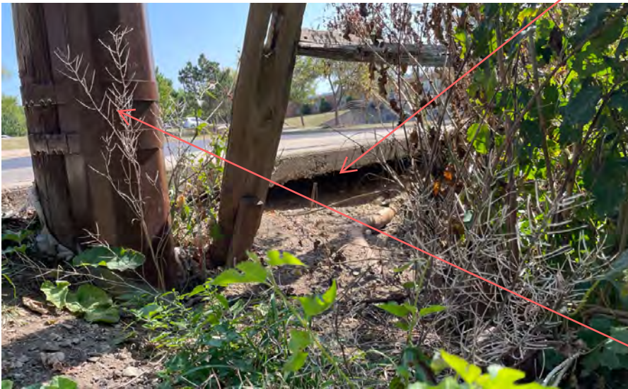
Photo 3 - Erosion causing undermined sidewalk & dangerous conditions
