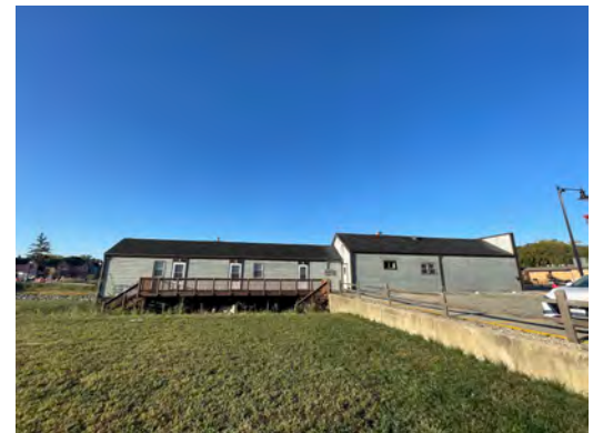
North side of building off Main St
