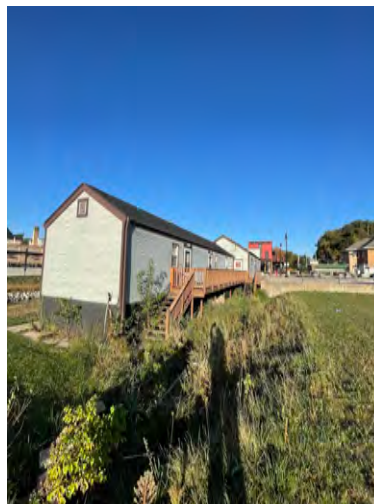
North side of building off Main St
