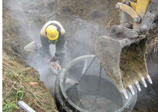
Streets crews work on installing a manhole
