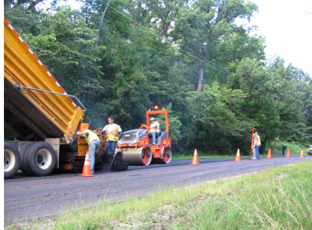
Public Works Department repaving Village roadway
