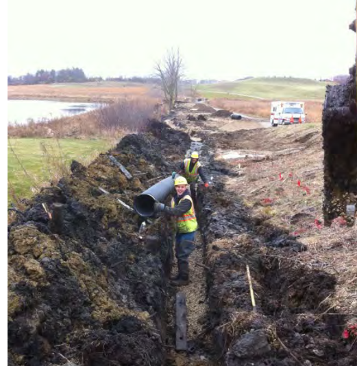
Village crews installing storm sewer drain
