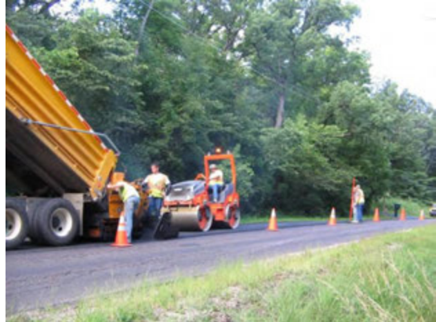
Village crews paving Highland Avenue
