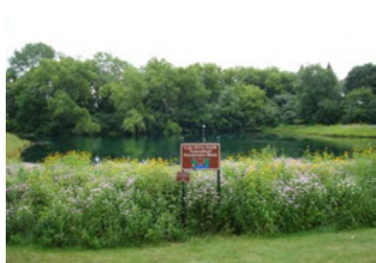
Arquilla Naturalized Stormwater Detention
