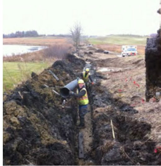
Village crews installing storm sewer drain
